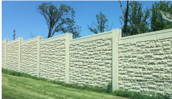
*Photo: example of pre-cast concrete with formliner*
